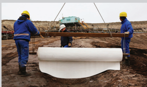
2- Construck Tex unrolling.
